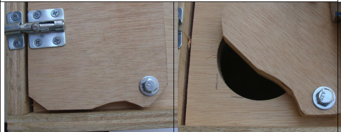
a. 1/8" gap around Door L/H & bottom side
